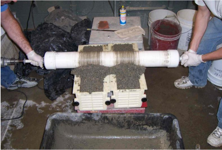
Figure 45. Finishing using a roller screed
