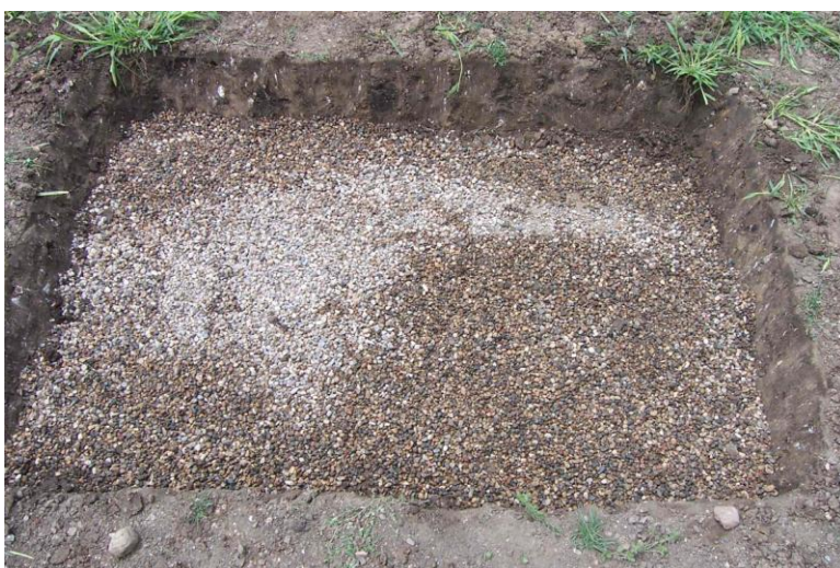
Figure 47. Aggregate base at test location
